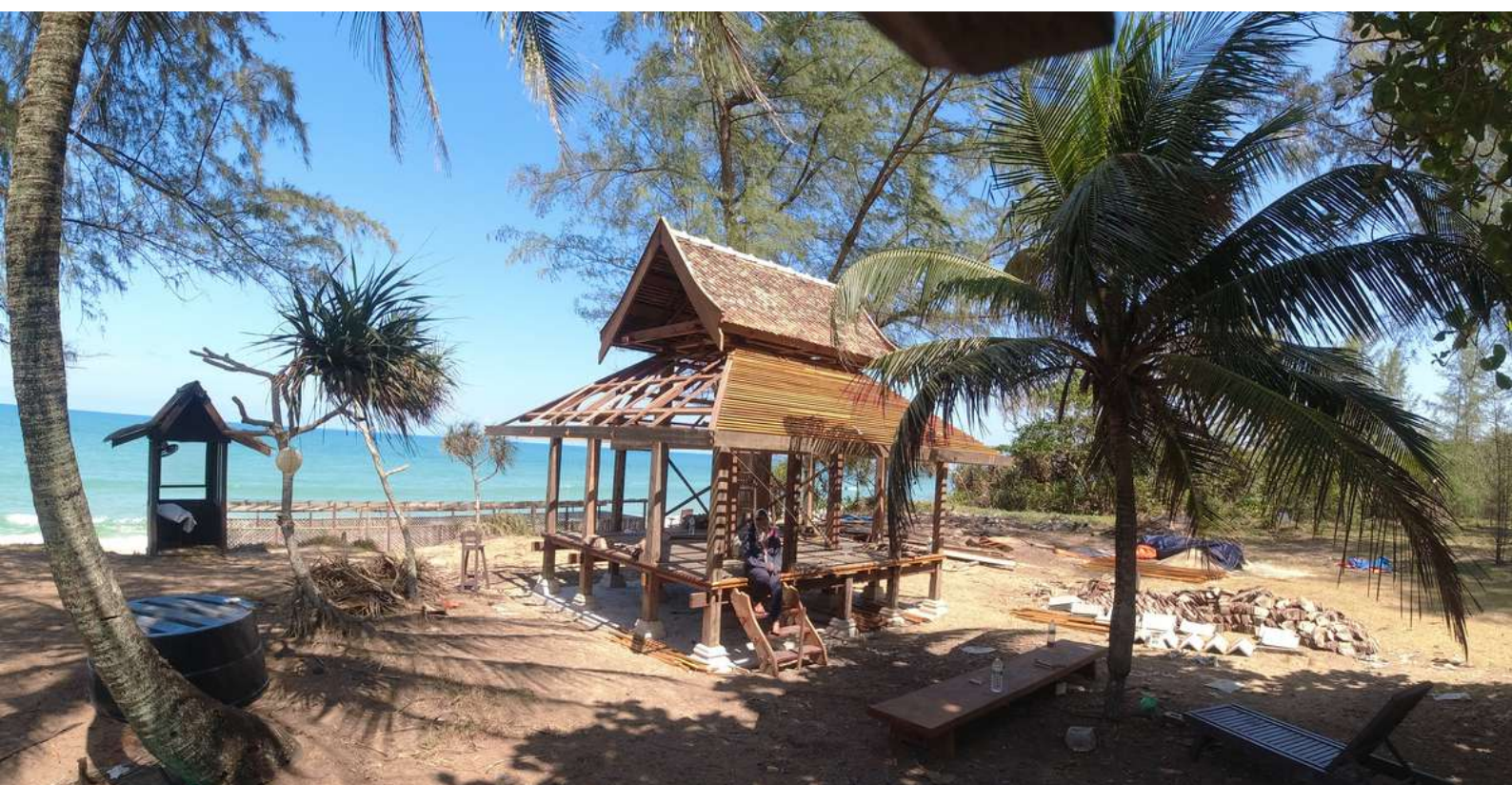
The construction of the new Visitors' Hut.
